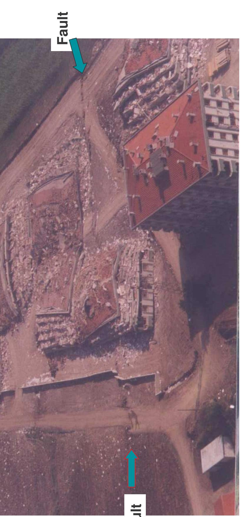
Izmit Earthquake  $M = 7.4$  (1999) – “Sandwich” failure of r.c. buildings
