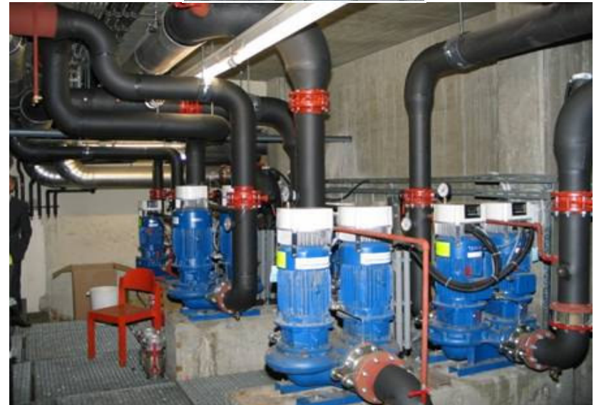
Heating circulation pumps Citytower, Vienna
