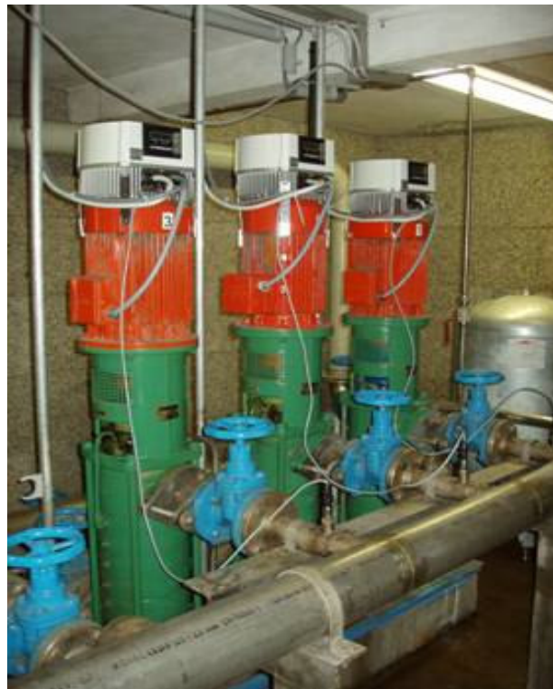
Water supply Klosterneuburg
