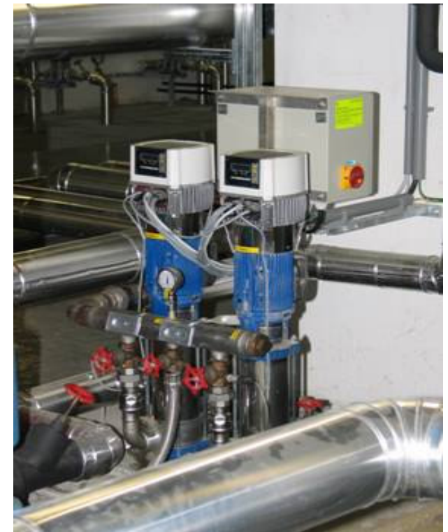
Booster system Hotel Hilton in Vienna
