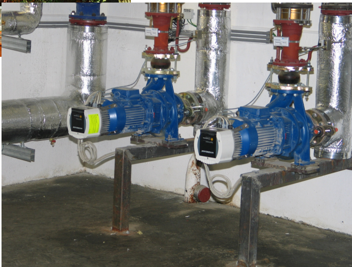
Heating circulation pumps Hotel Hilton, Vienna
