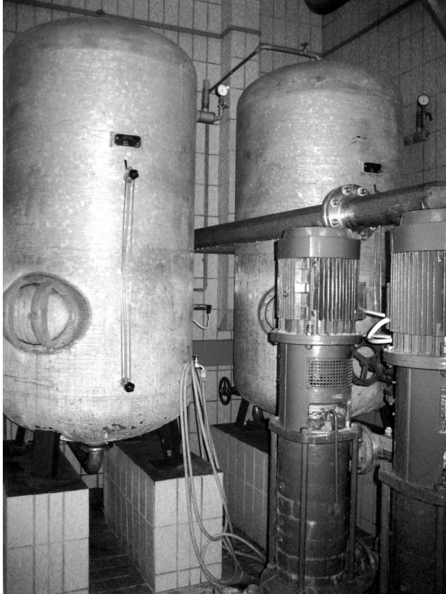
Fixed speed system with large pressure tanks and necessary air compressor
