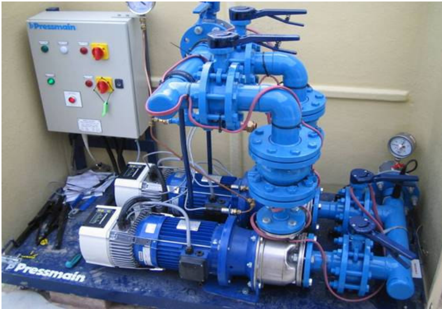
Booster set / Water supply Hunter's Lodge, UK
