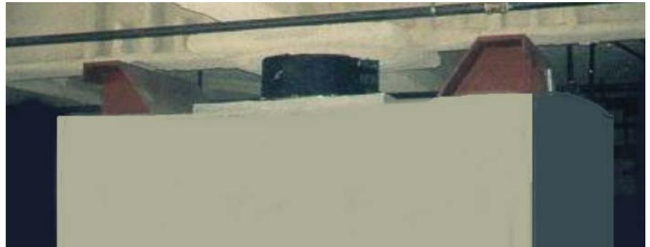
Figura 22. Fale-safe system verticale previsto per il San Francisco Emergency Management Center.
