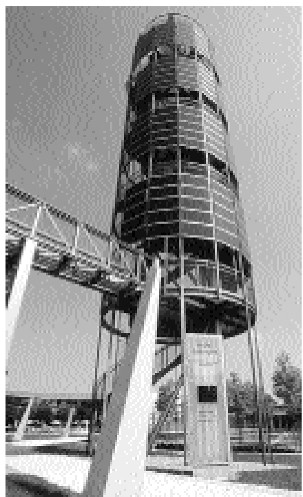
Fig. 21 Solar Tower, Heilbronn, Germania
